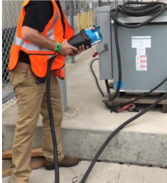
Figure 17. High Speed Charging Requires Large Diameter Cabling (TransPower)[19]
